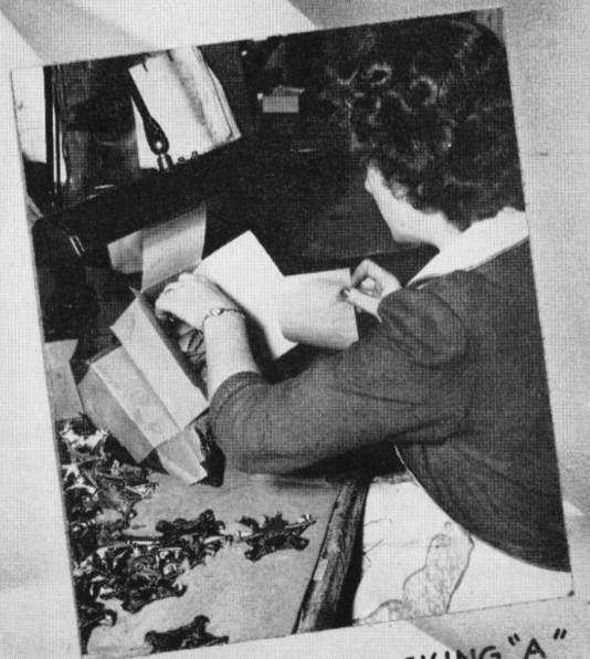
3. "MERRY CHRISTMAS" IS PIERCED INTO THE STAR IN PRESS No. 1. SALVATORA DIMARIA OPERATES THE PRESS.
