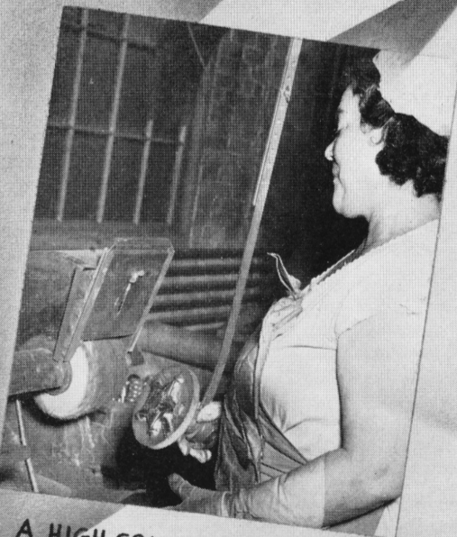
4. GIOVANNINA NANNI, ELECTRIC SHELL, TAPS THE BACKS OF THE ORNAMENTS FOR THE SCREWS WHICH WILL HOLD THE ORNAMENT TOGETHER.
